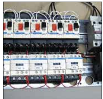
The electrical system is easy to service. The electric cabinet is located at a comfortable working height and all the components are clearly labelled. The system is carefully designed with a logical layout.
